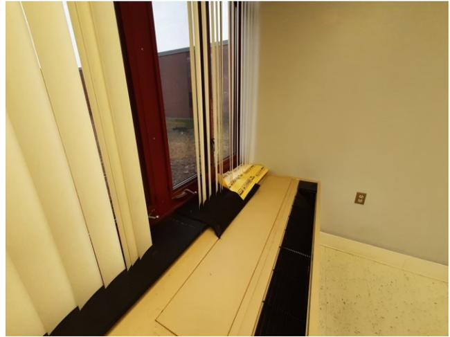
Photo 2: Classroom 128 - window leaks (note pads on window sill).
